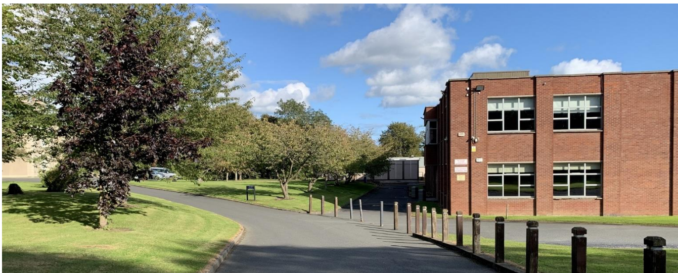
Plate 10.7 - View east along existing access to Sybil Hill House / St Paul's College. (New access road follows line of existing access road and passes through line of cherry trees in centre of image)
