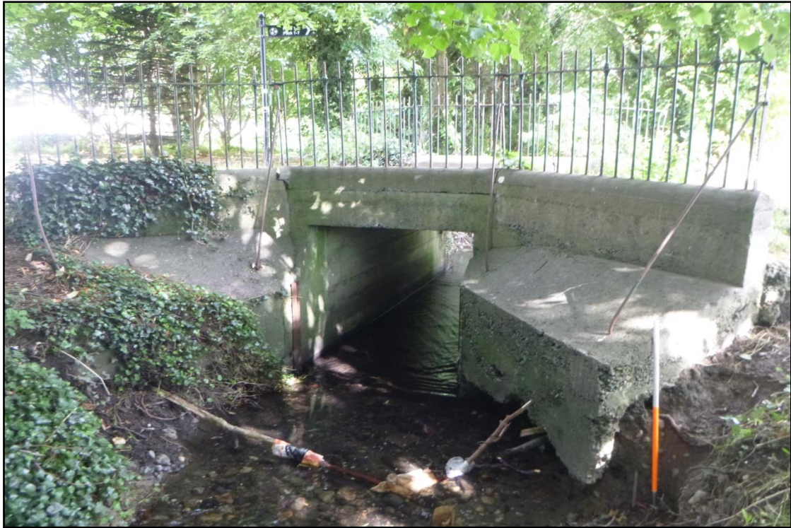
Plate 11-28: Concrete bridge with railing over Naniken River at entrance to St Anne's Park on All Saint's Road
