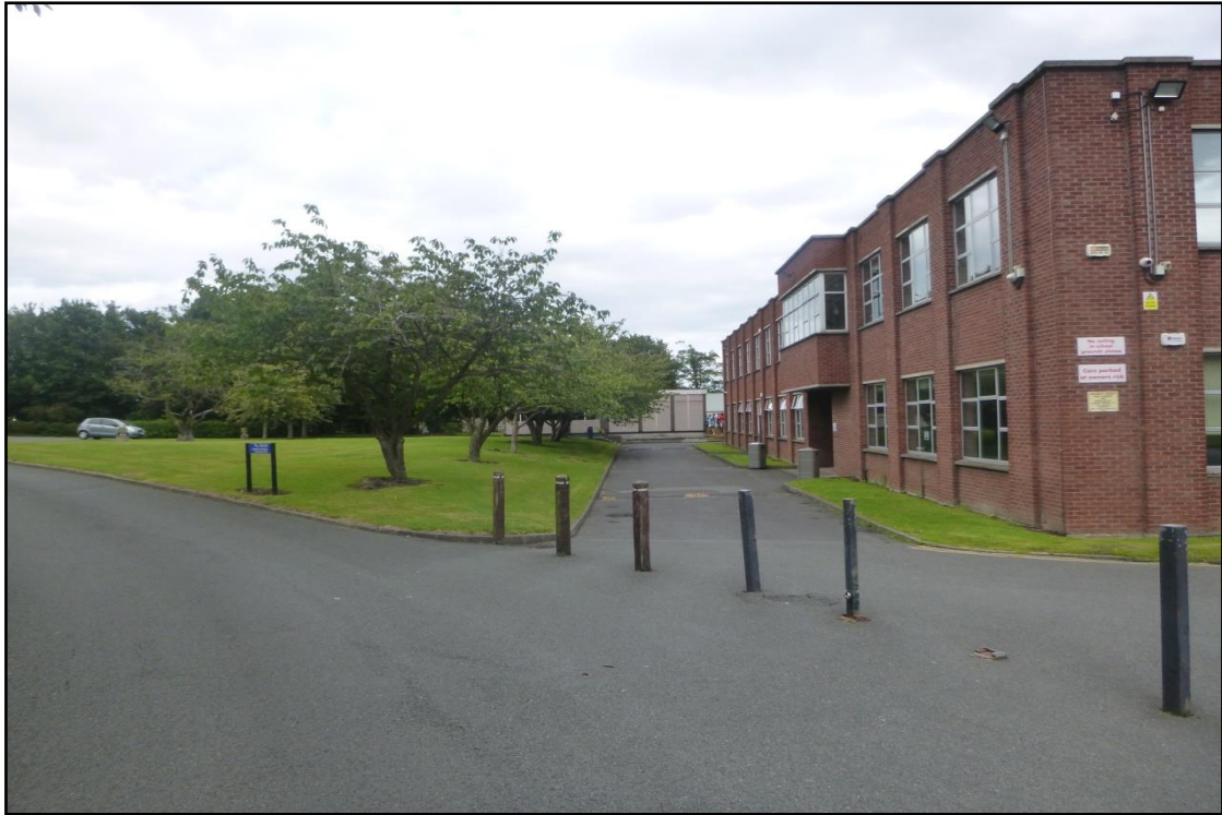
Plate 11-14: Existing access road between Vincentian Residence and St Paul's College at Sybil Hill House (AH2)
