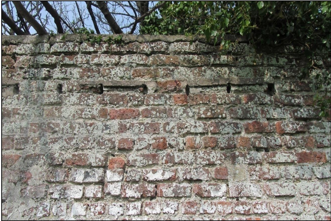
Plate 11.18: Detail of brickwork of extant garden wall (AH1). The remnant ridge of concrete and beam holes suggests a lean-to structure, such as a glasshouse, stood at this location
