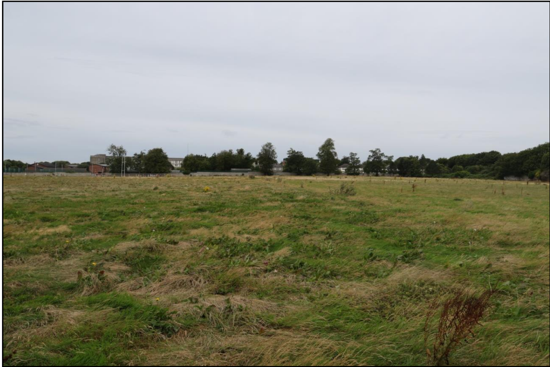
Plate 11-20: View west across Proposed Development site to Sybil Hill House (AH2) (at centre, beyond trees)
