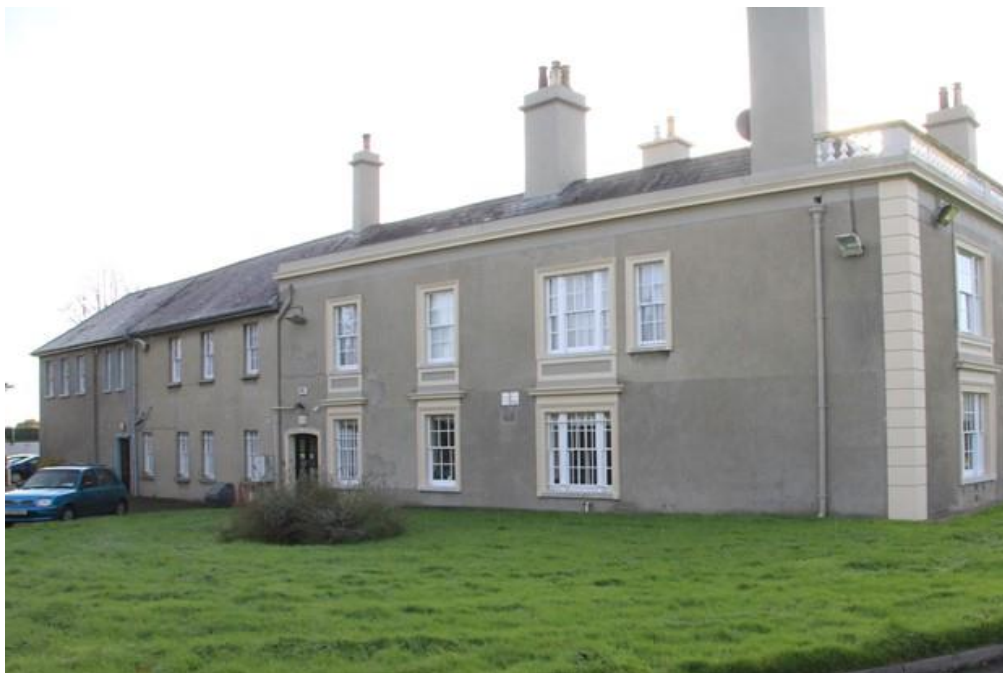
Plate 11-6: Northern elevation of Sybil Hill House
