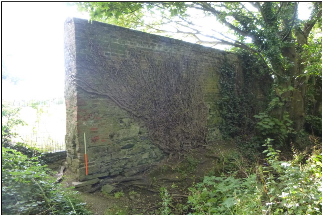
Plate 11.17: View south-west at rear east extent of wall of Maryville garden (AH1)
