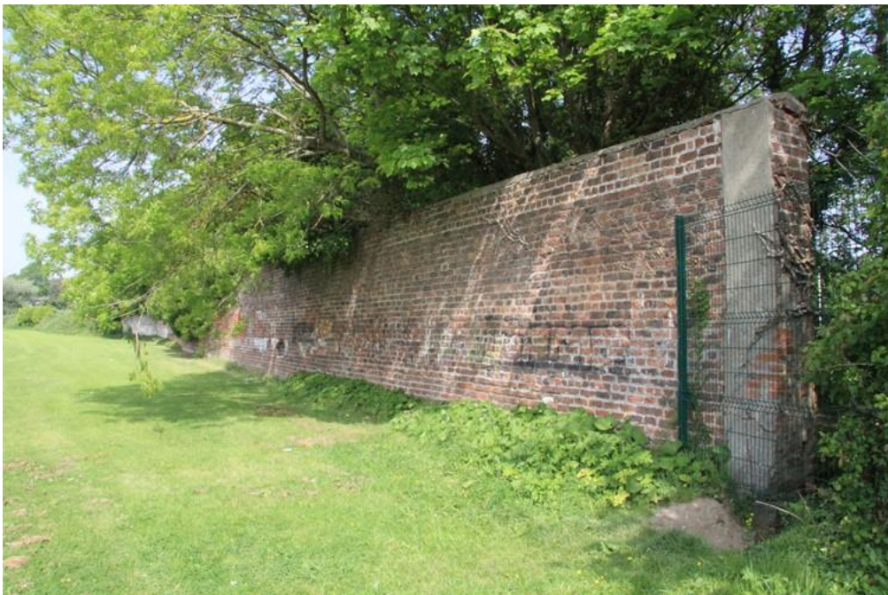
Plate 11-10: Brick-faced wall near the northern boundary
