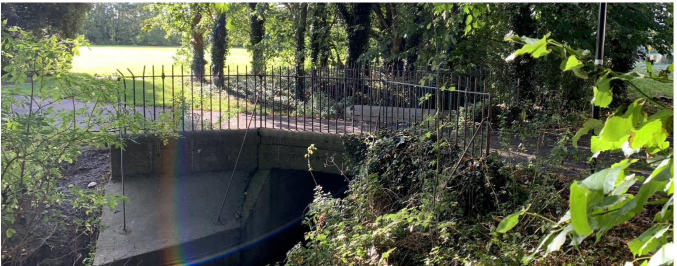
Plate 10.6 – Existing concrete and metal railing bridge over Naniken River
