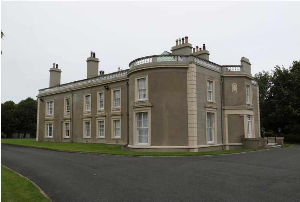
Plate 11-5: Sybil Hill House with southern elevation at right and western elevation at left
