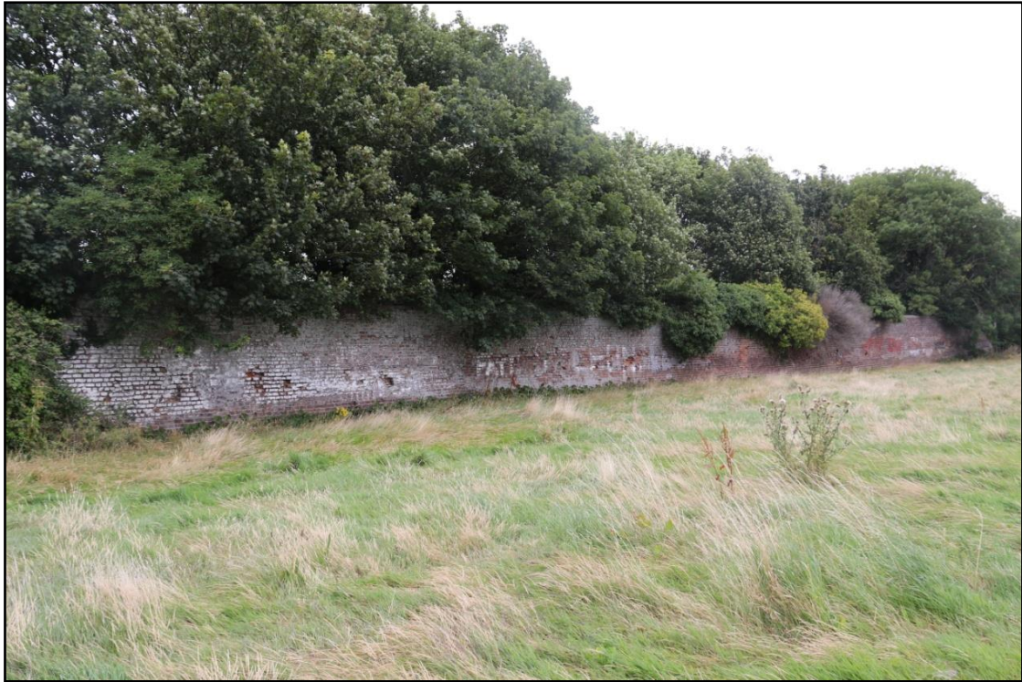
Plate 11-16 - View north-east along extant wall of Maryville garden (AH1)
